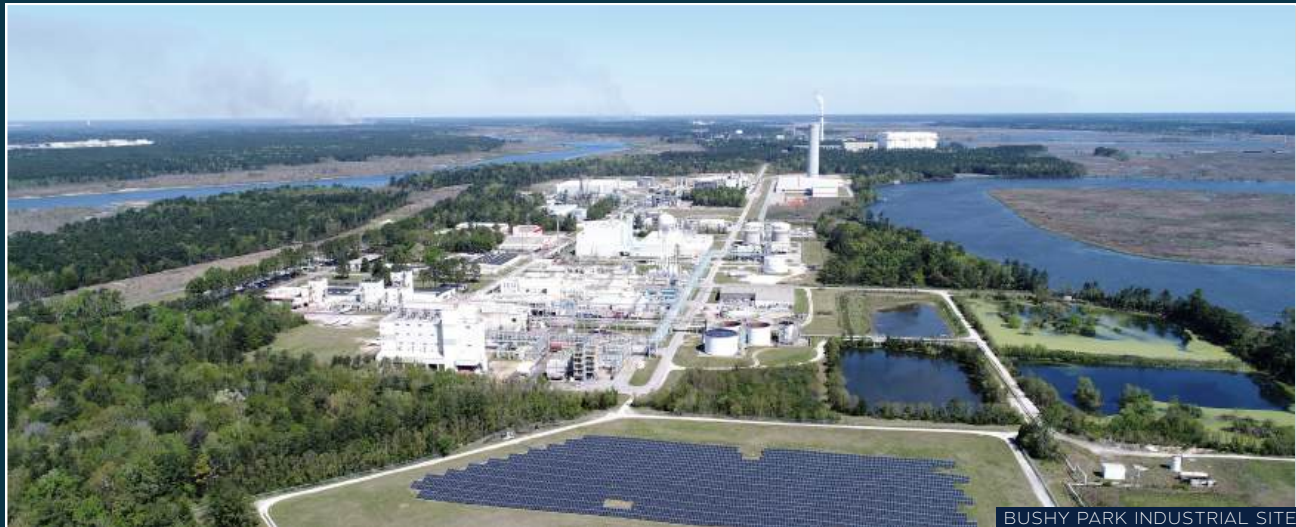
BUSHY PARK INDUSTRIAL SITE
